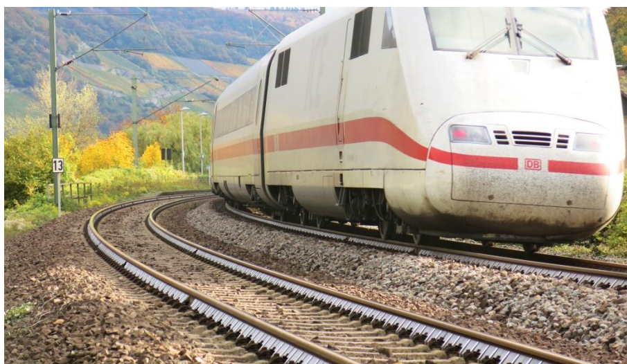
Figure 4 Calmmoon Rail project in Rhine valley – Germany
