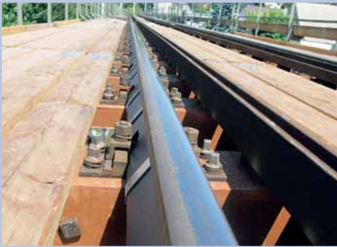
Fig. 3: Calmmoon Rail on a railway bridge with an open steel structure (source: the author)
