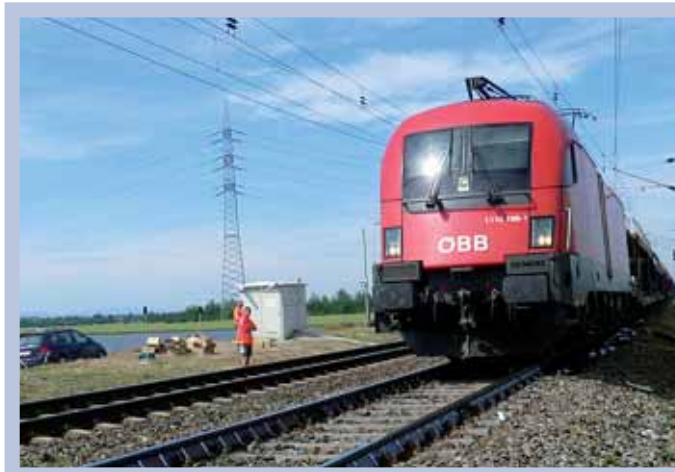
Fig. 1: Installing Calmmoon Rail on the test track in Deutsch-Wagram (source: Matsuda)
