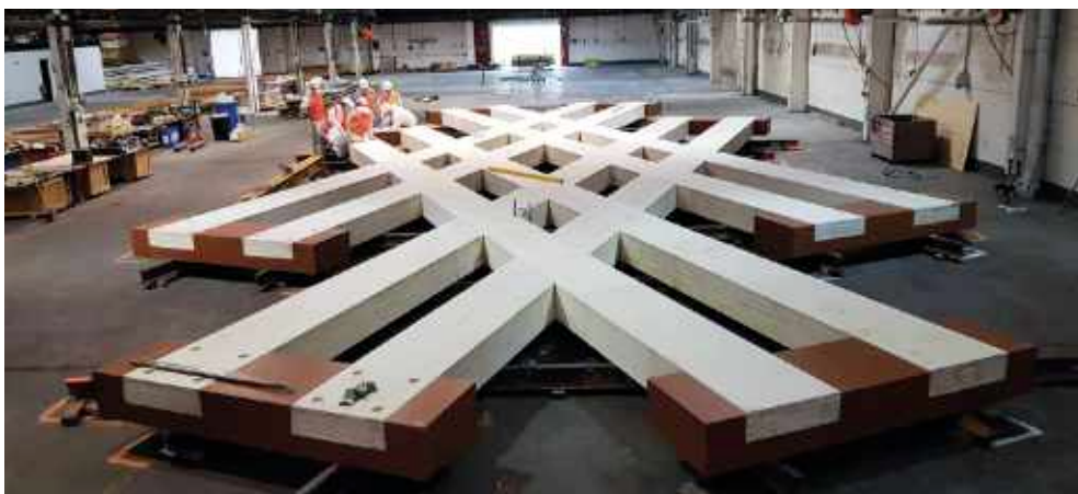
Top: The completed crossing was craned into position on August 26.
