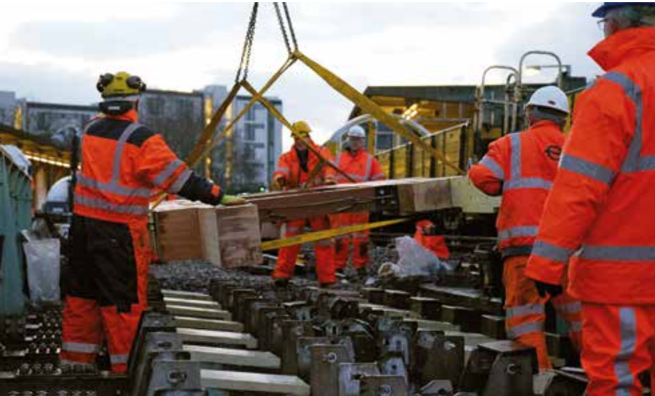
Sekisui FFU wedge packings installed to provide the required track cant when the longitudinal bearer frames are installed.
