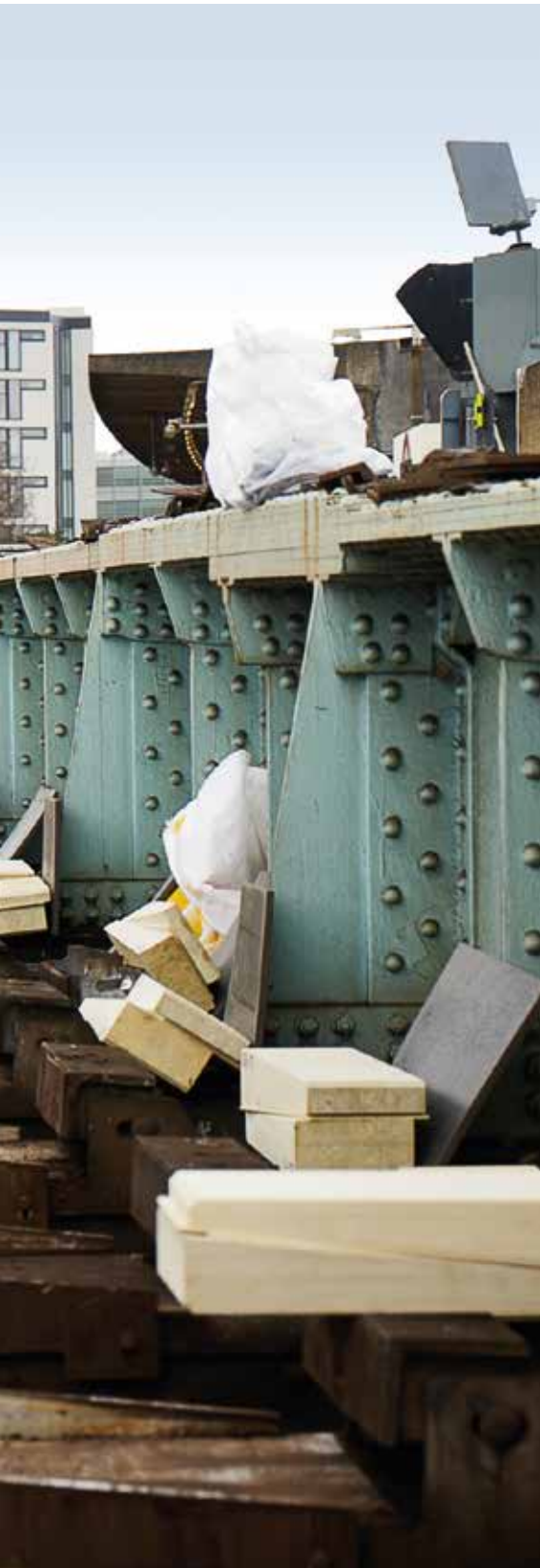
The prefabricated longitudinal bearer frames, manufactured from Sekisui FFU.
