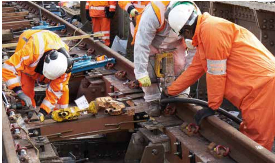
Longitudinal bearers, transoms and positive conductor rail blocks are all manufactured from Sekisui FFU. Here, baseplates are being secured.
