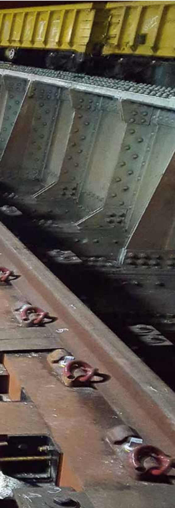
Longitudinal bearers, transoms and positive conductor rail blocks are all manufactured from Sekisui FFU. Here, baseplates are being secured.
